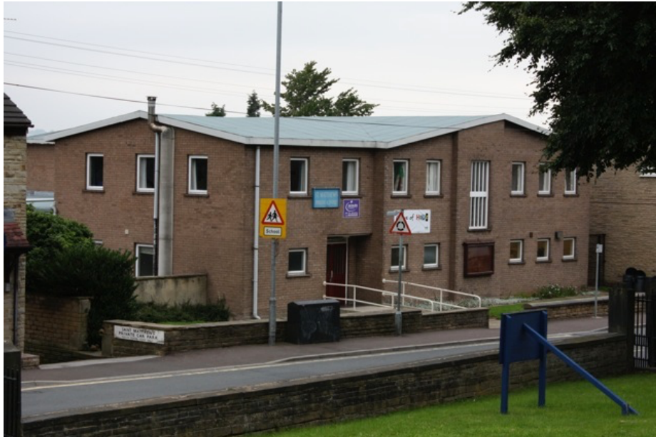
The Parish Centre with New Roof in August 2008
