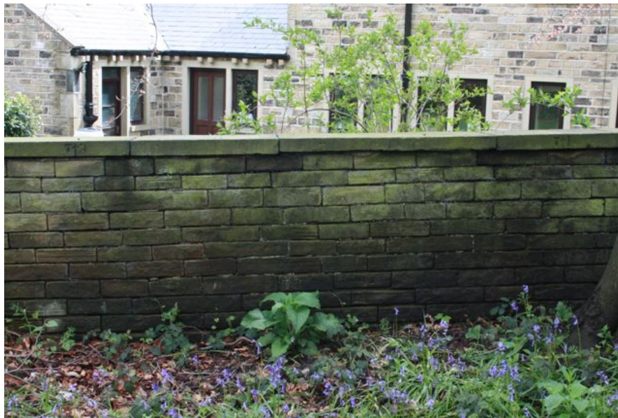
Churchyard East Boundary Wall adjacent 2 Vicarage Gardens
