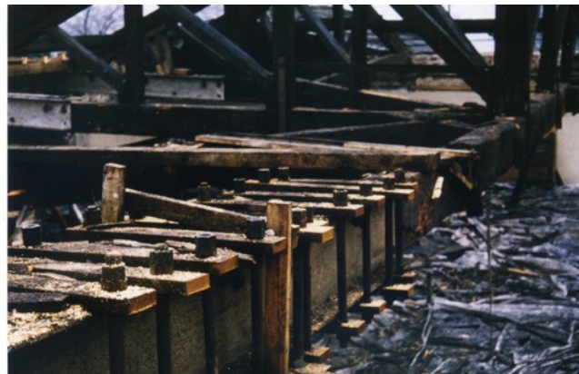
Straps and steel bolts on bottom chord of roof truss inserted in 1962/63 after Rentokil's work
