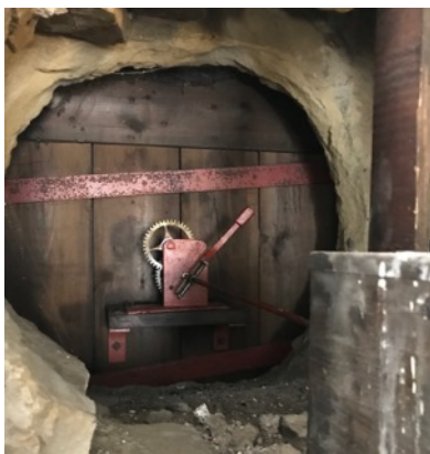
Refurbished dial works to west clock face
