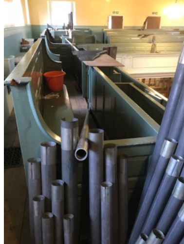
Dismantling and Cleaning of the Organ pipework
