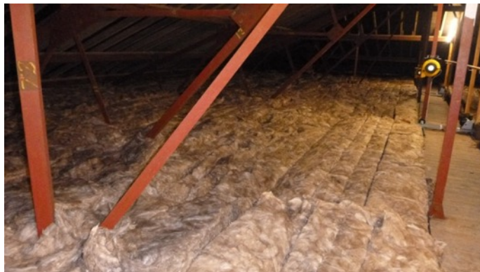
270mm Earthwool Loft Roll Roof Insulation above Nave Roof
