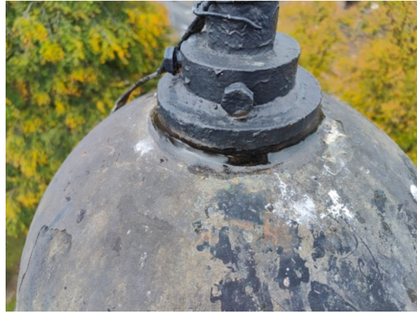
Sealing of weathervane to masonry Ball
