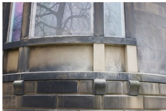
New Stones to Apsse Window Mullions
