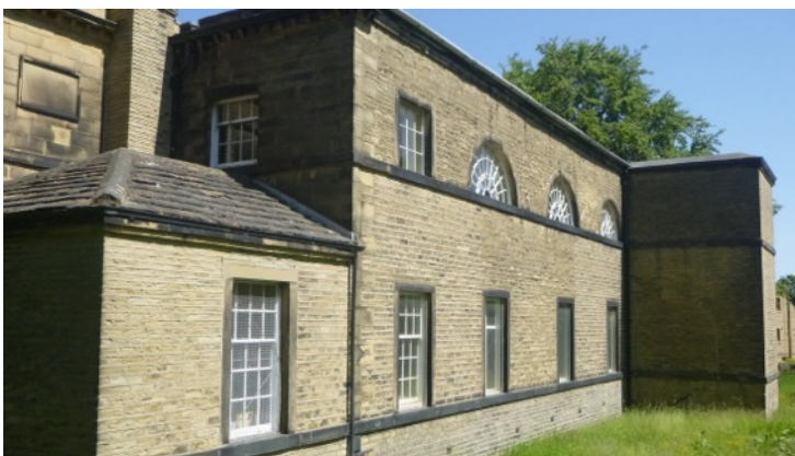
Repainted window frames on South Elevation
