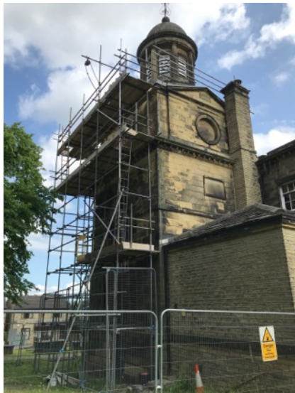
Scaffold to tower
