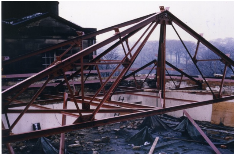
The new steel roof truss during construction in 1967
