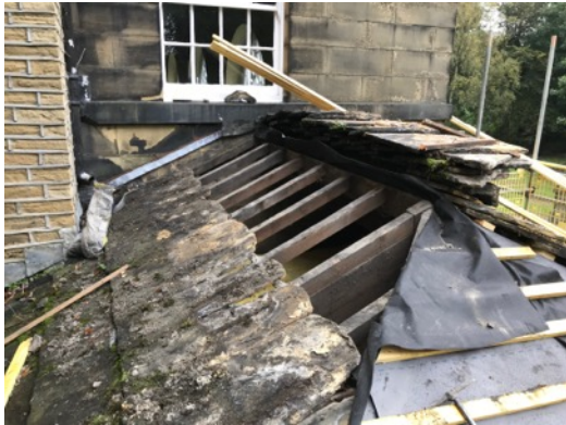
Re-roofing in progress
