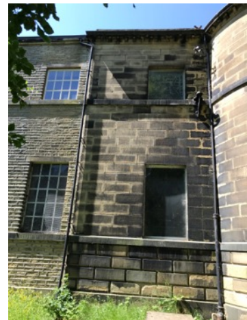
New window Frame installed (top left)
