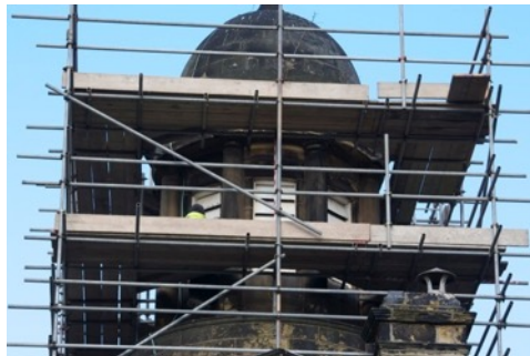
Scaffolding to Tower, 2010
