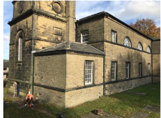
Re-roofing complete 18 October 2024
